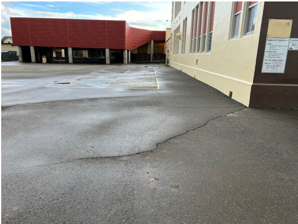
View from North to South on the North Side of Improvements
